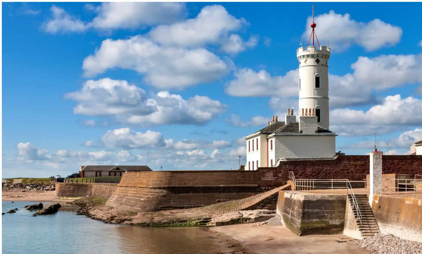
▲ Arbroath's Signal Tower. Photograph: John Bracegirdle/Alamy
